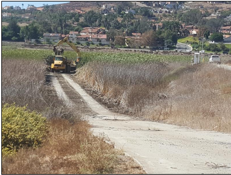
Accumulated debris and sediment are removed from a concrete swale at Hansen's Pond, an URDS facility.
