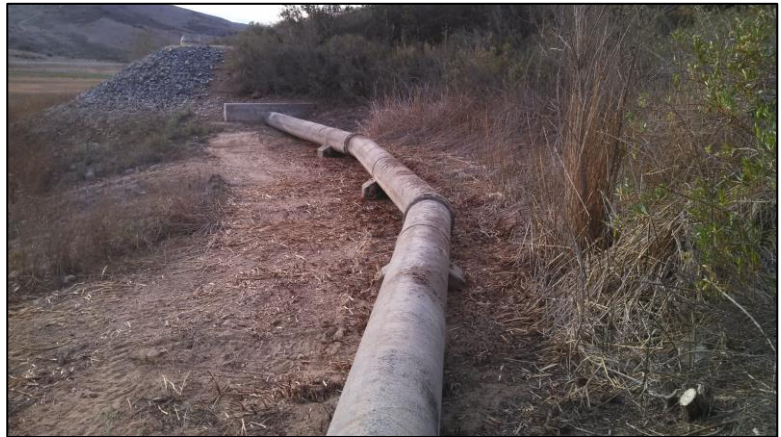
Many URDS facilities are maintained throughout the Sweetwater Reservoir property and the adjacent San Diego National Wildlife Refuge, including runoff diversion structures, supporting access roads, and drainage facilities.
