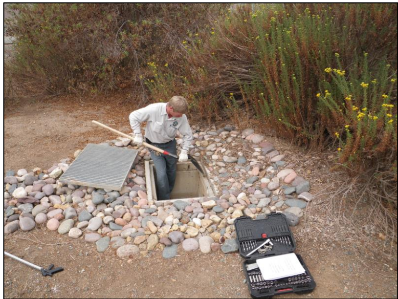
Stormwater facilities are maintained and repaired as needed. New facilities are installed as necessary to improve drainage and reduce impacts to water quality and hydrology.
