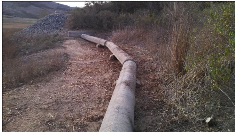
Many URDS facilities are maintained throughout the Sweetwater Reservoir property and the adjacent San Diego National Wildlife Refuge, including runoff diversion structures, supporting access roads, and drainage facilities.
