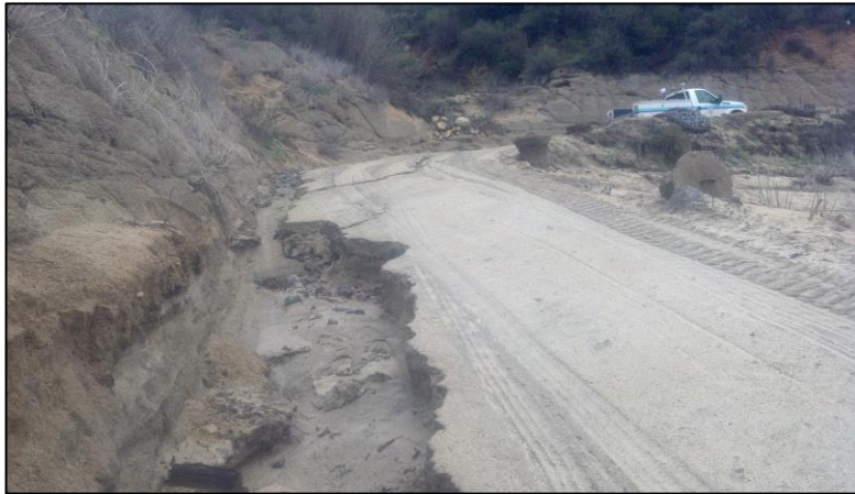
Erosion repairs may include a combination of short-term (e.g. re-grading) and long-term (e.g. installation of drainage facilities, paving, etc.) solutions.
